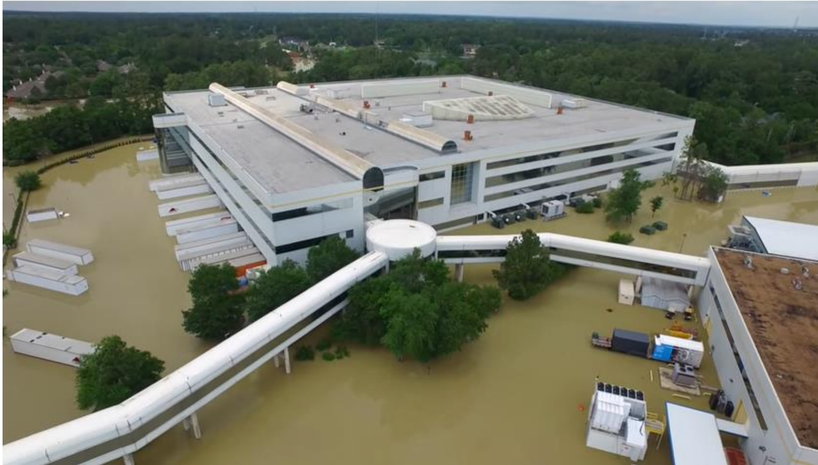
Hewlett Packard Campus along Cypress Creek, August 27, 2017.
